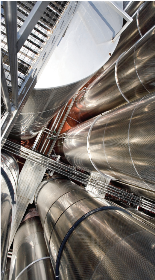
Silo, Tank and Hopper
